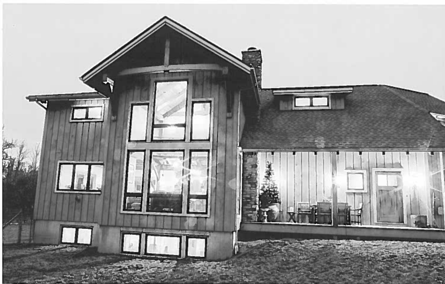
This Fairport home, built with Pioneer products, is conventional stick-built on the outside with a timber frame inside. MATT WITTMAYER
