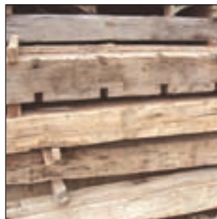
Original hand-hewn timbers
