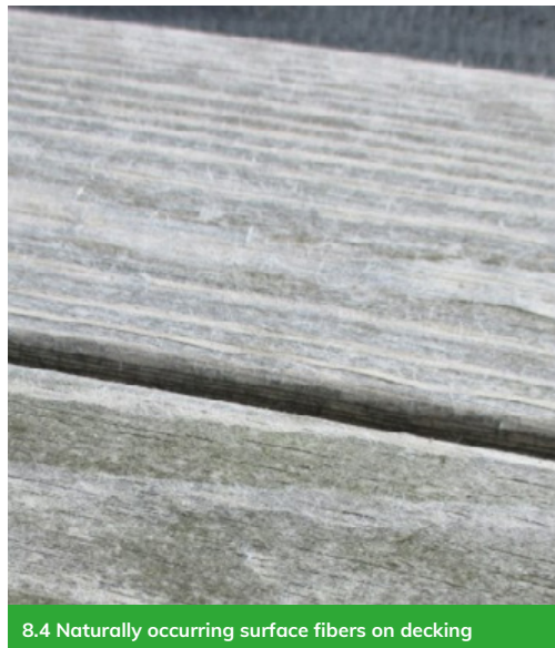
8.4 Fibers may get trapped in ribbed surface profiling
