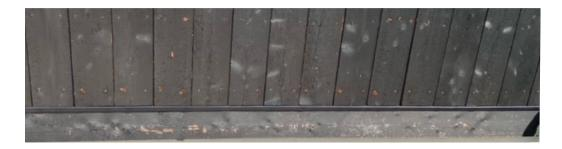
Over-driving fasteners and aggressive material handling during installation will result in a scarred surface where the char layer comes off, revealing the lighter wood underneath. Shown on Larch Deep Char.
