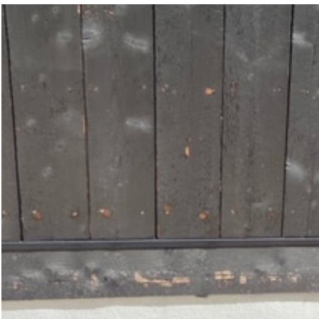
Bright wood exposed due to over-driving of fasteners. Shown: Larch Deep Char.
